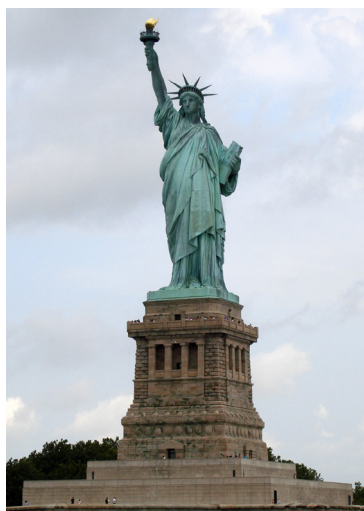
The Statue of Liberty is green due to oxidation of the copper sheets from which it is made
