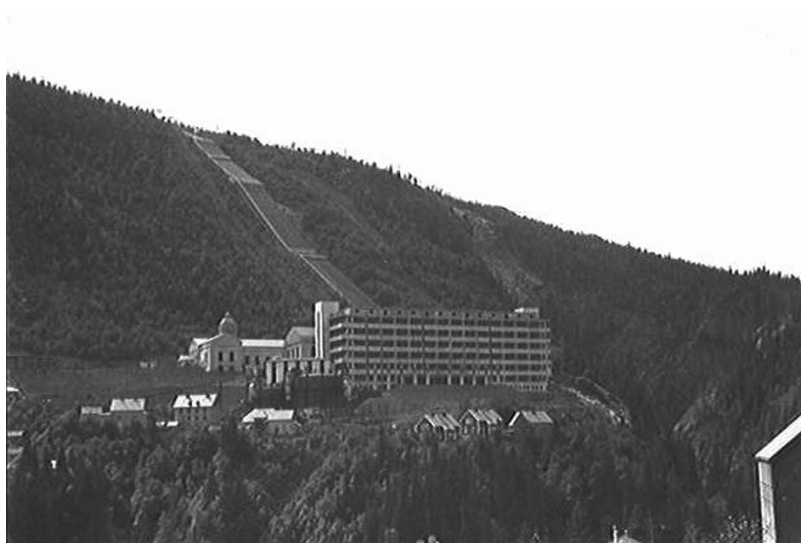
Vemork hydroelectric power station at the Rjukan waterfall in 1935
